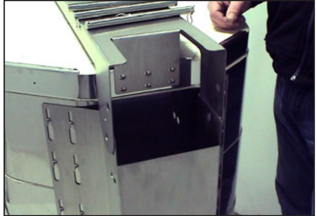
The Lid as ready for Hinge installation:
