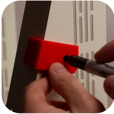
Making a mark for drilling.
