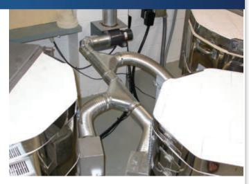
This shows several small kilns hooked up with one Vent-Sure using two Vent-Doublers.
