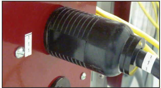
Element jumper cord properly installed:
