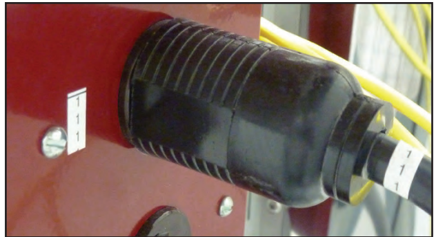
Element jumper cord properly installed:
