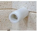
thermocouple from damage while loading. Also any metallic flakes from the thermocouple will tend to drop inside the tube where they can be vacuumed out during normal maintenance. (hotkilns.com/ protected-thermocouples)
