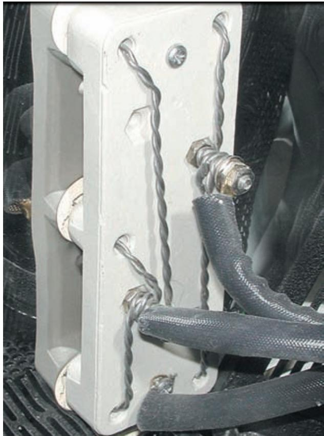
Proprietary all-ceramic element connection block makes changing elements easy. Terminal hardware allows you to get good contact with the element with minimal effort. ([hotkilns.com/ceramic-terminal](http://hotkilns.com/ceramic-terminal))
