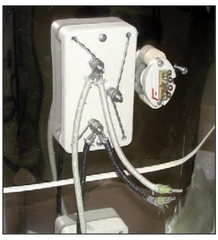
A close up showing how all the terminals of the wire and terminal hardware go together (shown before being tightened). Be sure to tighten this well because a loose connection could cause overheating at the terminal:
