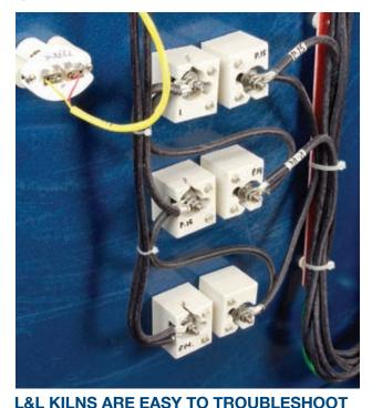
Open up any L&L kiln control panel and see how easy it is to check amps, element resistance, and voltage. No other kiln can be serviced as quickly, easily, or inexpensively as an L&L kiln.
